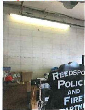
ACM wall texture in upstairs restroom
