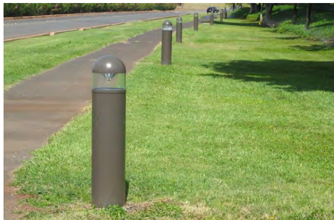
Solar photovoltaic trail lighting
