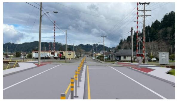
**Planning level cost opinion:** An order-of-magnitude planning level cost opinion was prepared for the median barrier on OR 38 based on unit costs from similar projects in the Pacific Northwest. The cost opinion accounts for design and construction along with several other factors. Potential right-of-way and property costs are not included at this time. The cost opinion is \$400,000.
